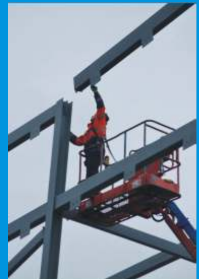
A workman carefully lowers one of the steel girders into place.
