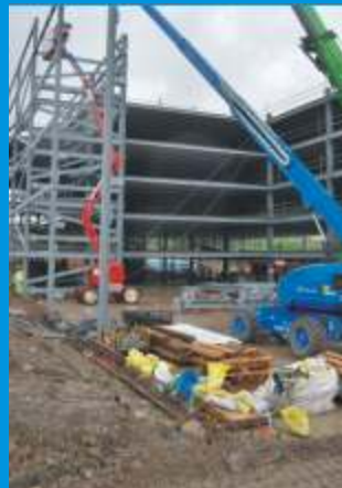
The new staff car park starts to take shape.
